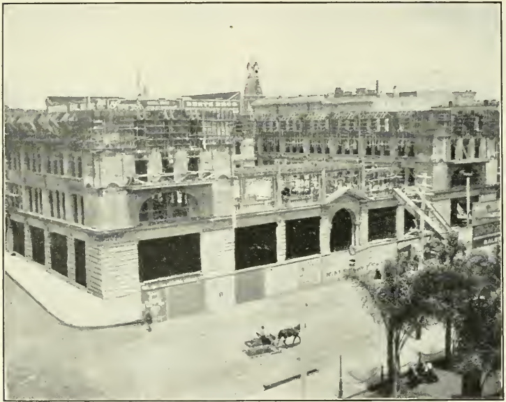
U. S. GRANT HOTEL IN COURSE OF CONSTRUCTION, JUNE, 1907
